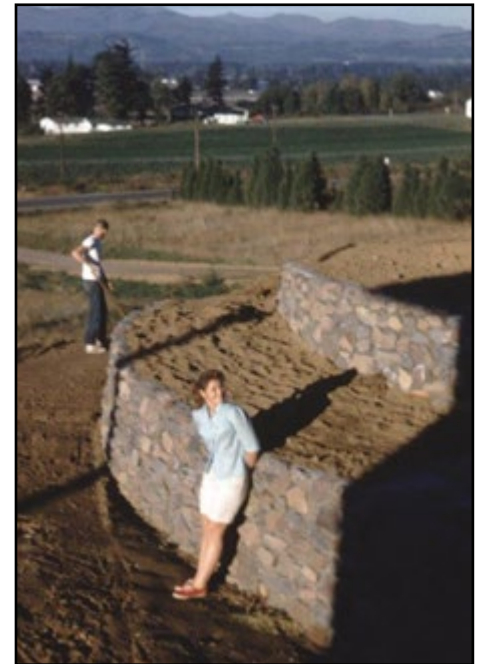
Handy House, 1959 - new rock retaining wall Bonnie Blough and Dale Handy, students of Reynolds High School, later marry
