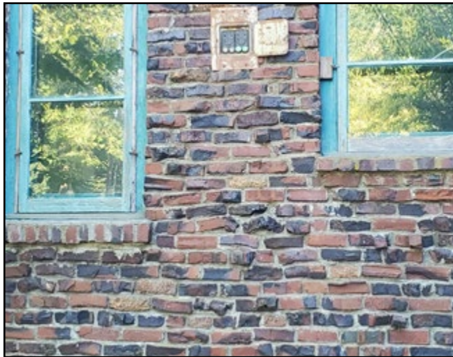
Clinker Bricks on Bondesson House, August 2021
